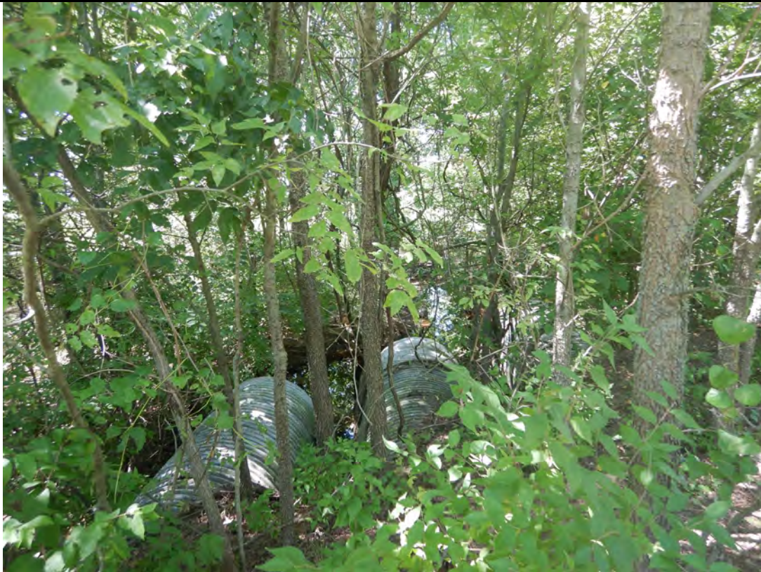
Photo 12: View of a triple pipe culvert approximately 500 feet west of Wetland 2. A channel is present on the south side of the track in this area, outside of the study area. Facing southwest.
